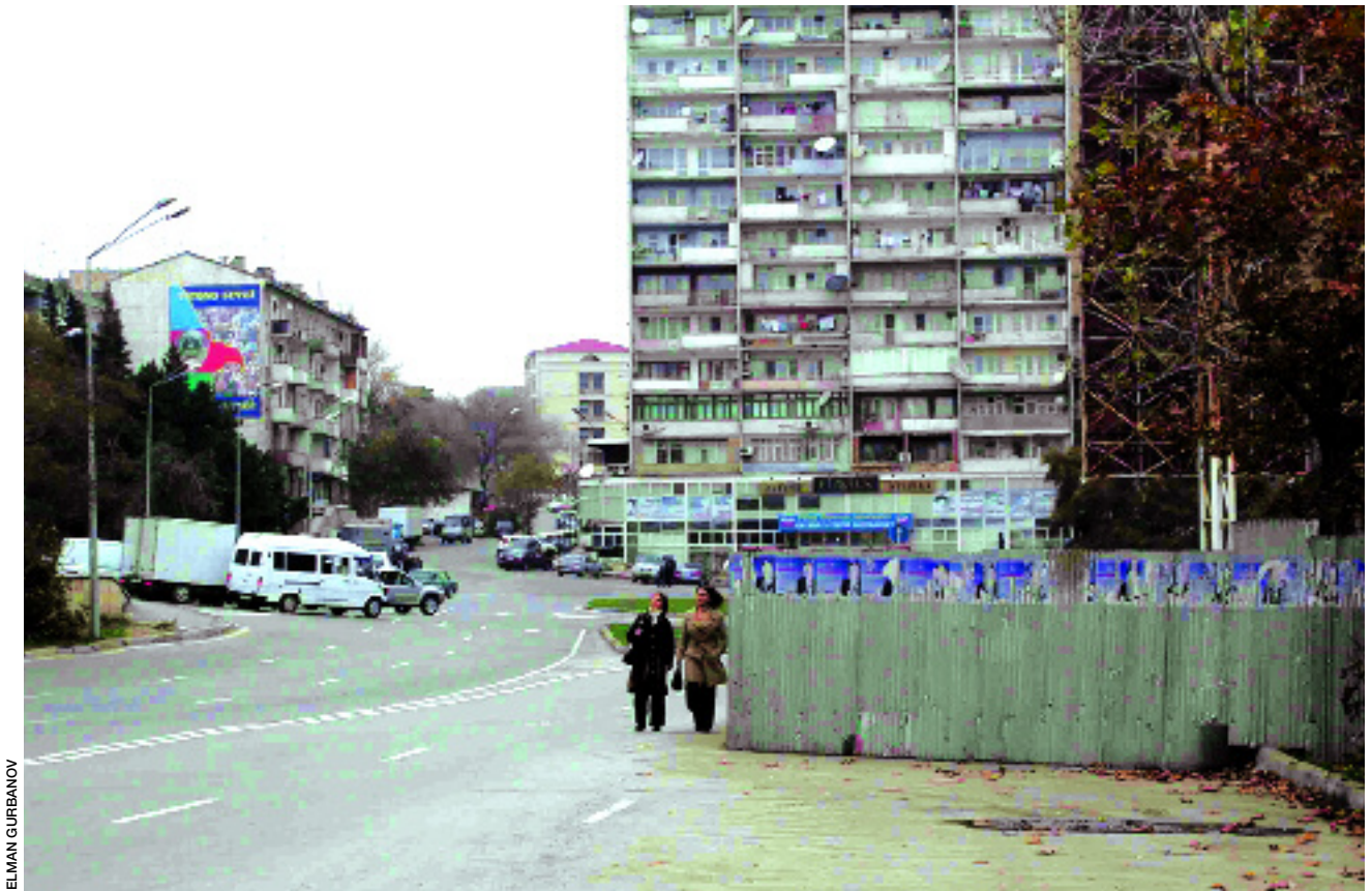
A frequent practice in Baku is to build a fence around the construction site that protrudes far out into the street (see top corner on right hand page and photo above). This obstructs public space and creates enormous traffic congestion. Techniques and methods exist for handling tight urban sites which do not intrude into public space but yet ensure the safety of pedestrians and the flow of traffic.
