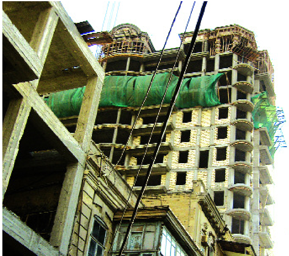
Heavy limestone blocks are commonly used as construction material in Baku as a substitute for lighter weight bricks or blocks (see blocks in the wall partitions in the high rise). The use of limestone blocks is extremely dangerous under seismic conditions. The abrupt lateral force of an earthquake will cause any wall without steel rebar reinforcement to collapse. This is the most common cause of death in earthquakes zones.
