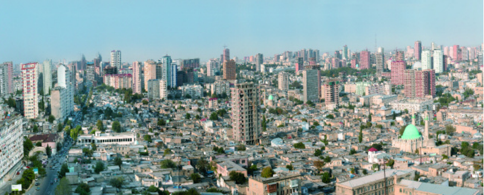
Panoramic view of Baku's skyline. More than 500 towers have been erected in the past five years. Architecturally, there is no sense of unity and cohesiveness. Photo: Pirouz Khanlou, October 2005.
